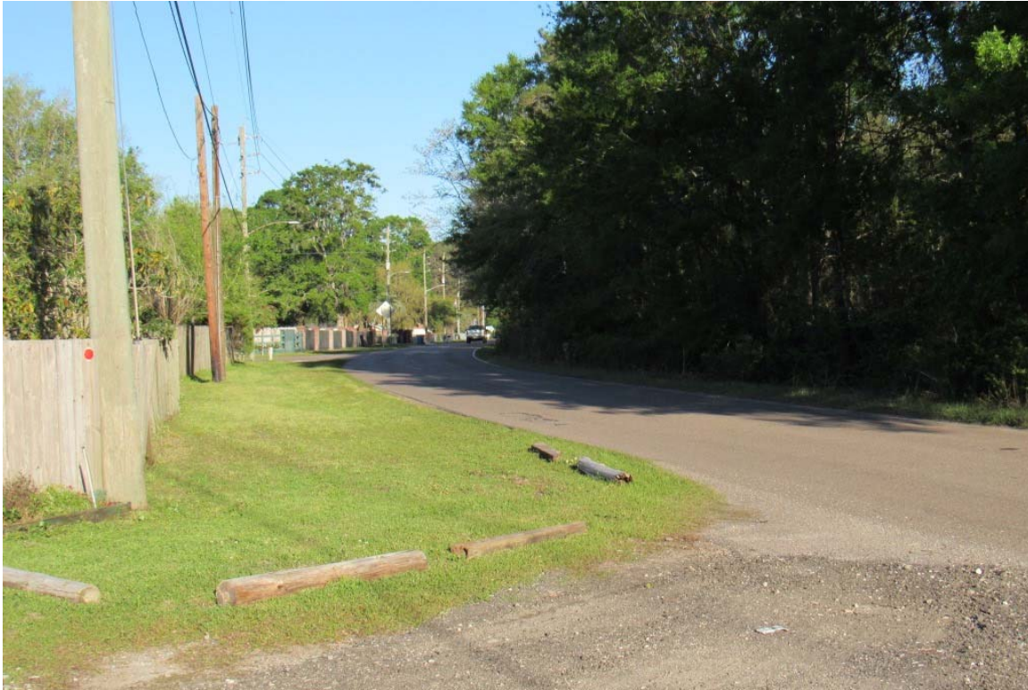
View along Duval Road. Subject property is on right side of photograph
